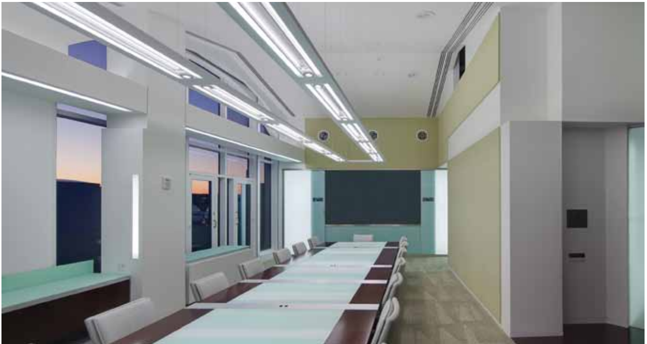
A structurally complex ceiling made it challenging to achieve necessary illuminance levels in the boardroom. A direct/indirect pendant provides 30 vertical and 75 horizontal footcandles over the boardroom table, and dimmed T5s supplement vertical illuminance between the table and the video monitor.
